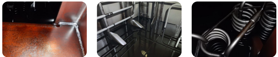
Figures 5, 6 & 7: No sludge deposits from VLSFO tanks after 4 months using Aderco 2055G
